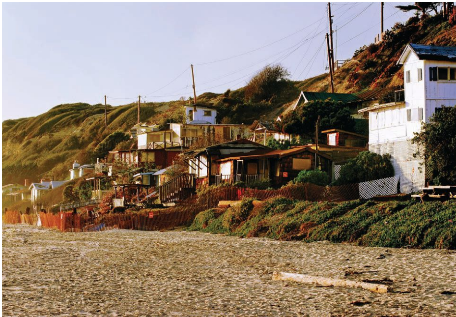
Seventeen cottages await restoration on the North Beach.
